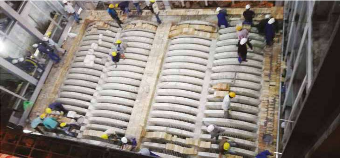
Rider Arch Construction at site
