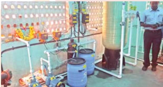
Installed new RO Iron removal plant at Thiruvottiyur Plant
